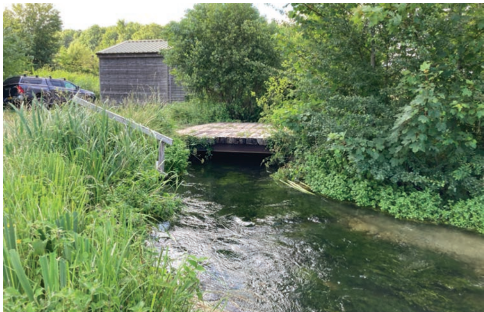
Narrow bridge at the entrance to Abbotts Barton
