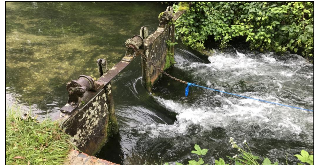
Weir & hatches: obstruct fish passage & reduce upriver flow - increasing siltation
