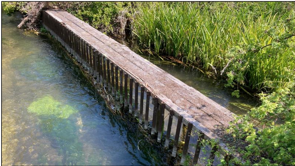
Weir & hatches: obstruct fish passage & reduce upriver flow - increasing siltation
